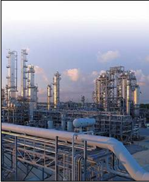
Huntsman's Port Neches Plant
